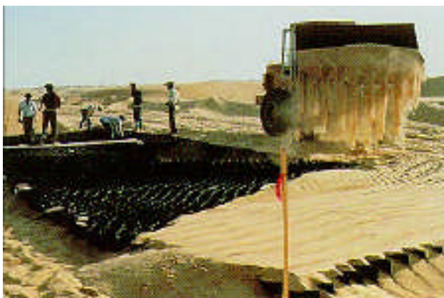
Photo 5-4: Sand filling of geocell by front end loader
