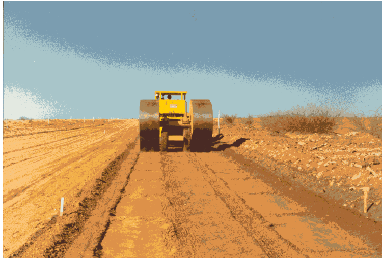
Photo 6-1: Compaction of subgrade/fill by impact compactor
