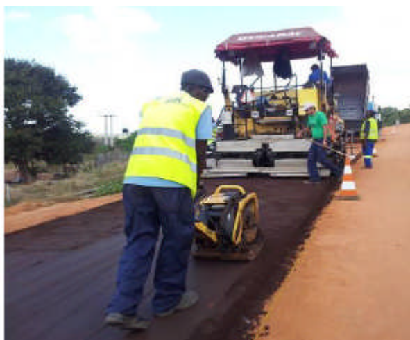
Photo 5-3: ETB construction-plant based approach
